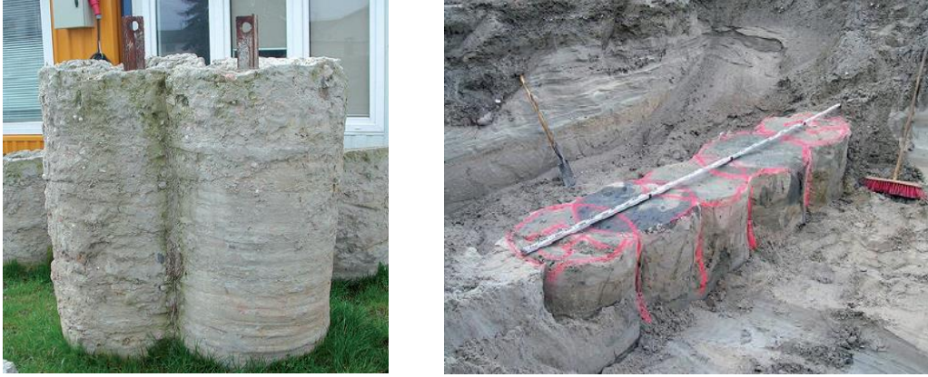
Figure 1: Exposed cut-off wall with secant DSM columns: Courtesy: Keller, Deep Soil Mixing [1].
